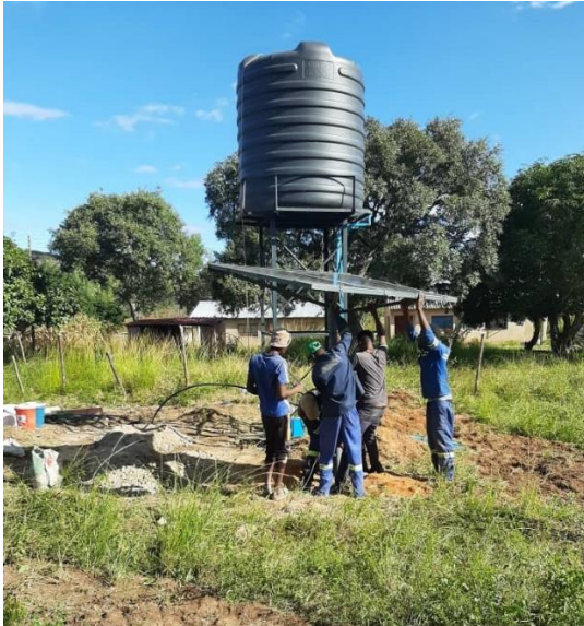
Contractors installing solar water system
